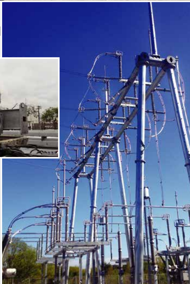
Prototyping Assy and Shipping of a 138kV Wide Flange A-Frame
